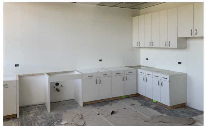
Level 2 Casework Installation
