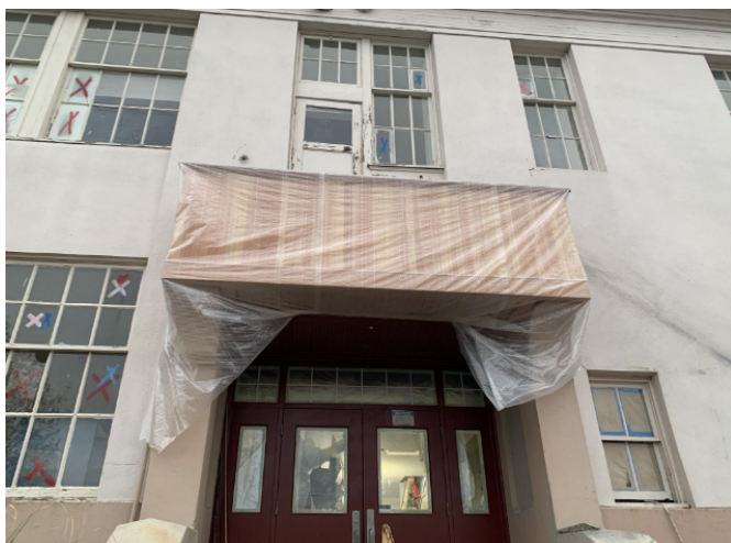
West Balcony Exterior Framing
